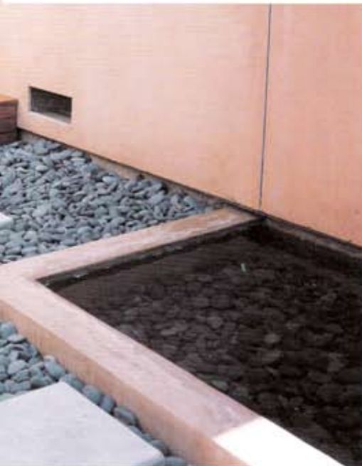
Inner Entry Court at Ensley Avenue
